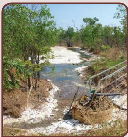
Fig 1. Mine drainage Photo: SKM
