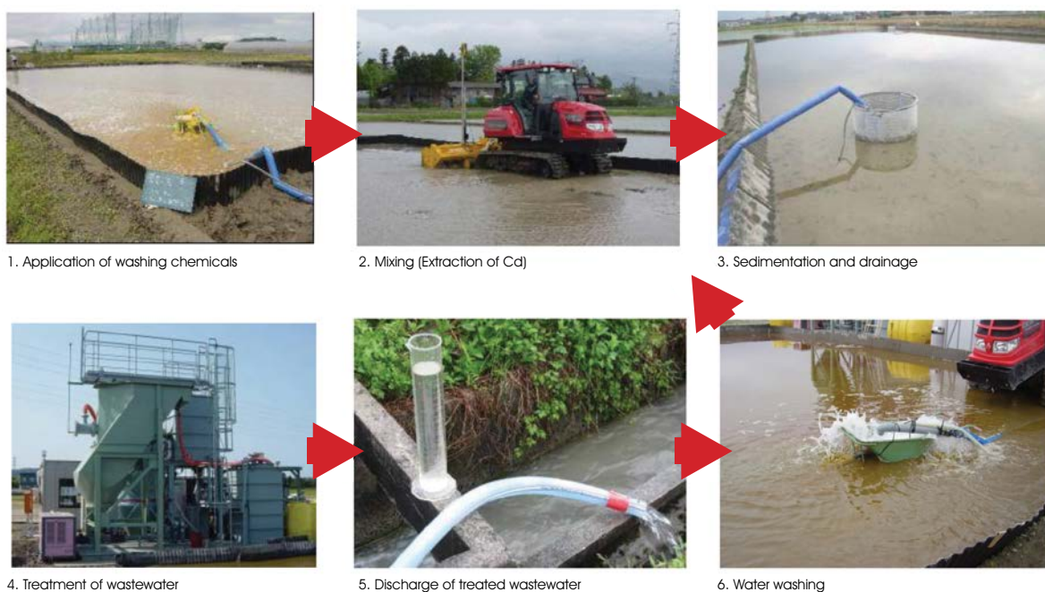
Figure 2. On-site process of soil flushing
