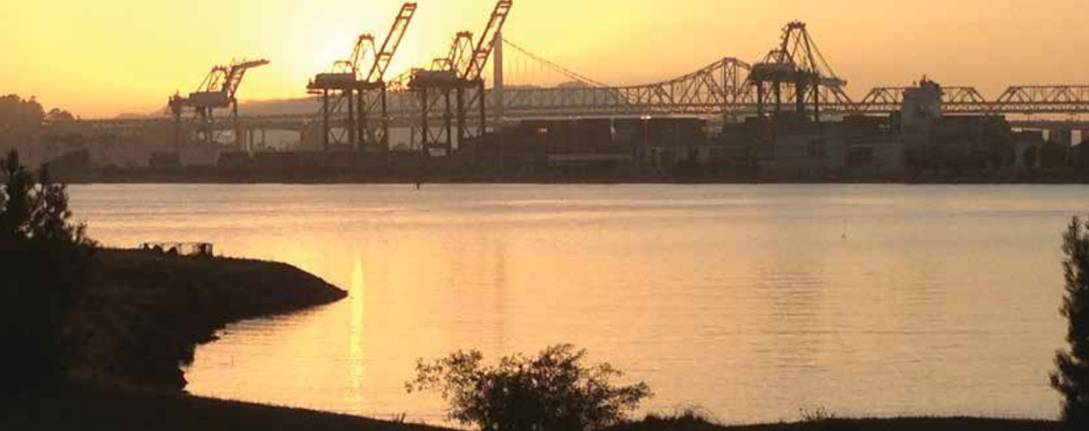
Remedial efforts at industrial areas near shorelines will be prone to sea level change considerations.
