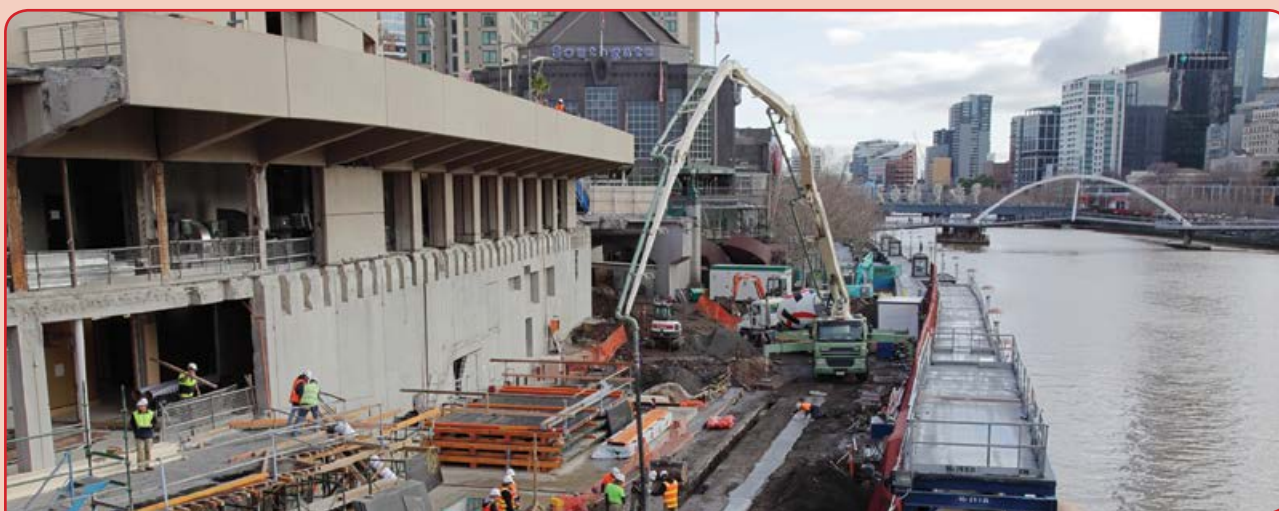
Construction on the Yarra River in Melbourne.
