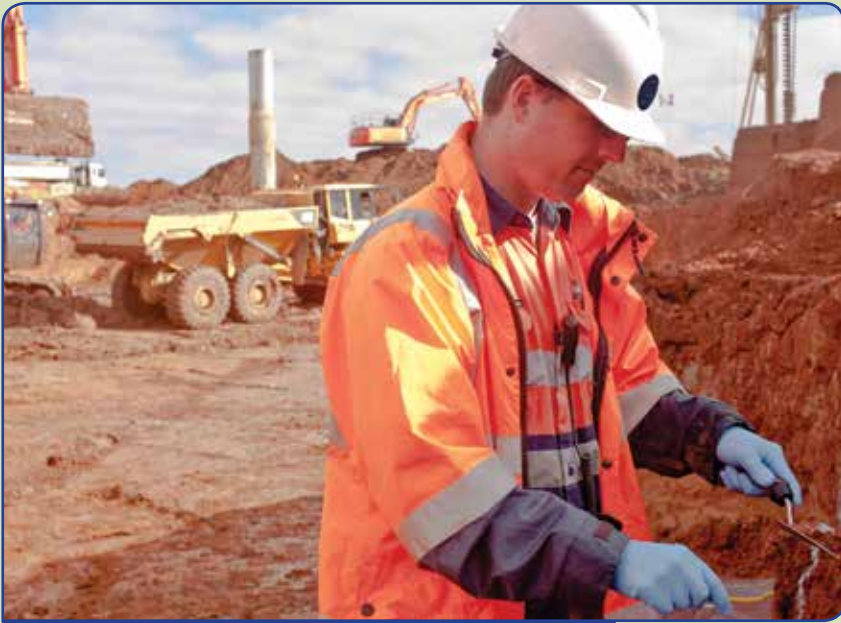
Remediation works at the site of the new Royal Adelaide Hospital. FMG Engineering.
