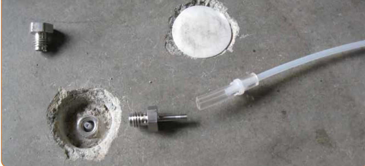
Preparing to sample for sub-slab vapour intrusion. Photo courtesy of author.
