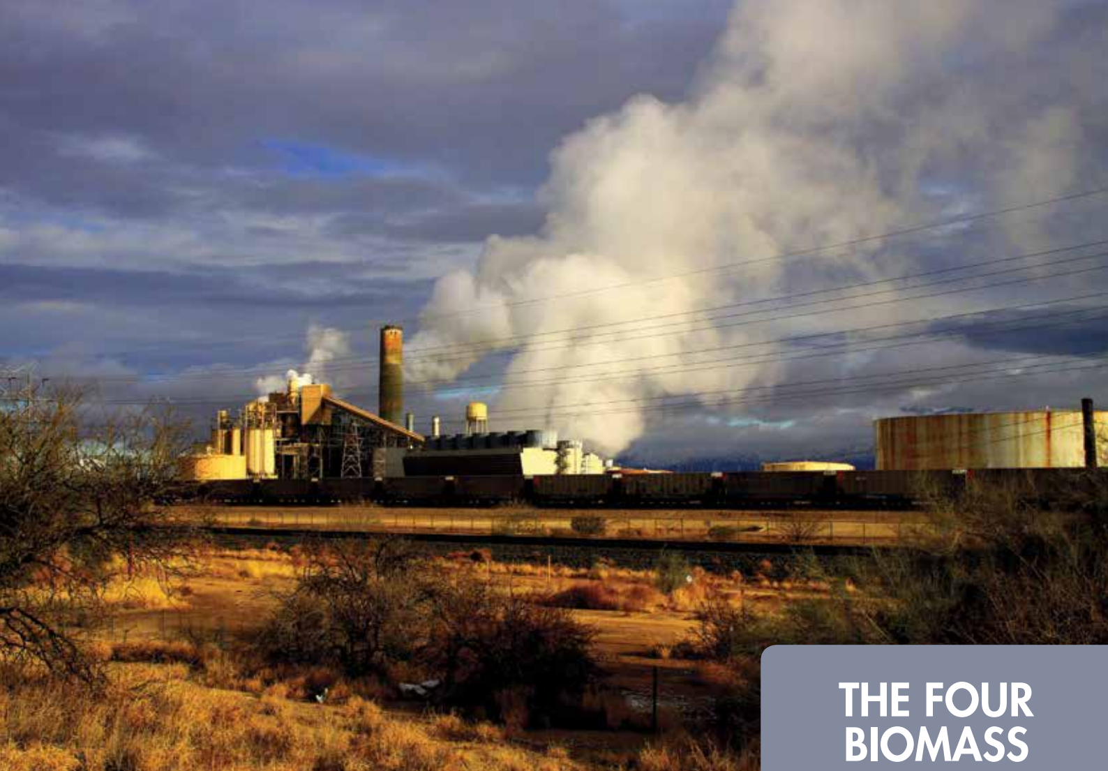
FIGURE 1 Irvington Generating Station. Operated by Tucson Electric Power, the station produces electricity by fossil fuel combustion. The fuels used consist of coal, natural gas, liquid fuel and landfill gas. SOURCE Bill Morrow http://bit.ly/FlickrBillMorrow
