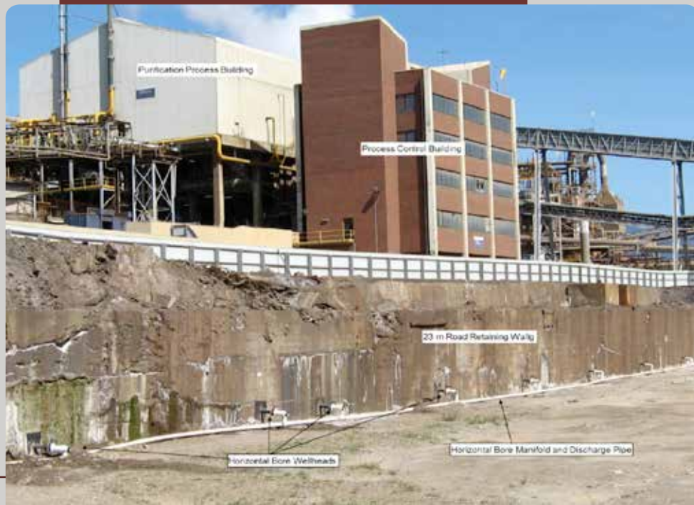
FIGURE 6 The finished bore manifold at the base of the retaining wall.
