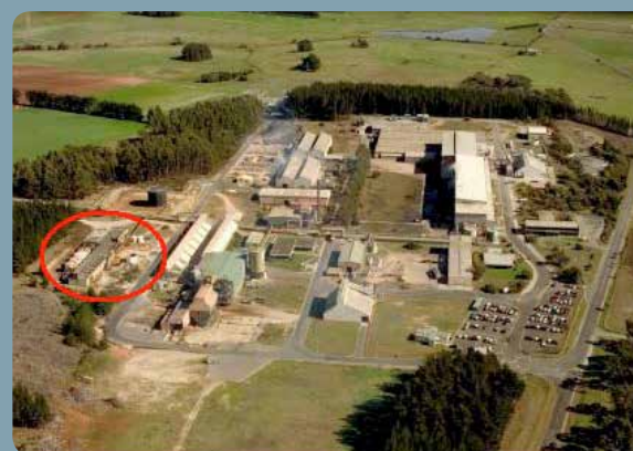
The Wesley Vale Pulp and Paper Mill, showing the location of the chlor-alkali cell plant
